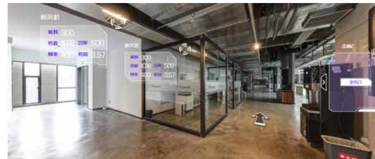
360 Panoramic Display and Control of Office Area HVAC
